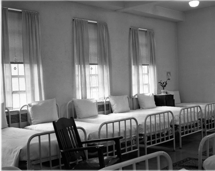
Figure 3 - Old hospital dormitory (Ann Arbor News, 1937)
